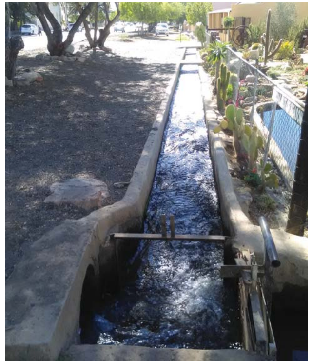
Prince Albert town leiwater system passing in front of Zwartberg High School.
